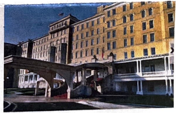
The French Lick Springs Hotel features a spa, casino and many activities for children. A hotel has been on the site since 1845; part of this building dates to 1901.
